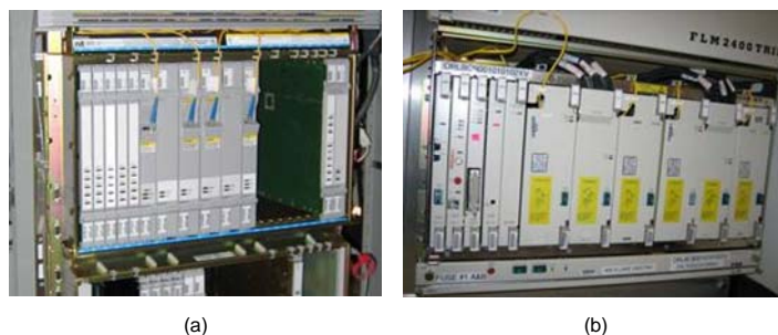
Fig. 2 (a) Nortel Optera 3500 and (b) Fujitsu FLM 2400 SONET systems
